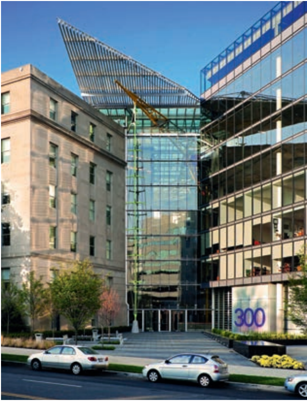
Büroobjekt America's Square, Washington, D.C., JAMESTOWN 29 / JAMESTOWN Premier
