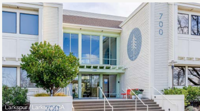
Larkspur / Larkspur, CA
